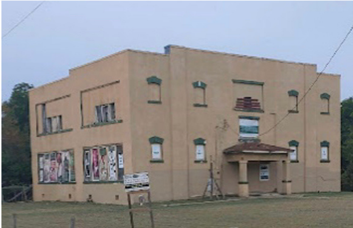
Vocational High School built in 1923 was once occupied by Royal Feast Masonic Lodge #214, Most Worshipful Prince Hall Grand Lodge of Texas
